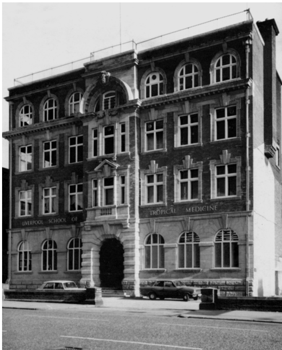
Façade of the Liverpool School of Tropical Medicine (1975). MILLER (1998), p.32.
